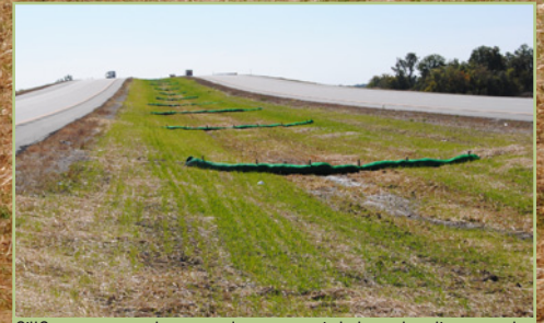
SiltSoxx were also used as area inlet protection and check dams.
