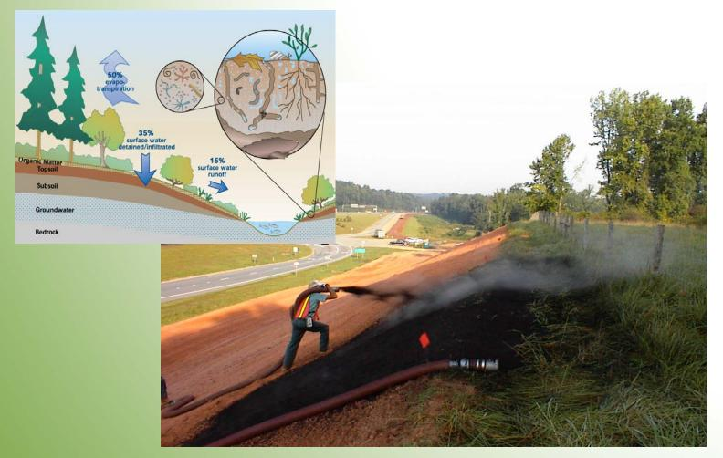
**Designed to:** 1) dissipate energy of rain impact; 2) hold, infiltrate & evaporate water; 3) slow down/disperse energy of sheet flow; 4) provide for optimum vegetation growth
