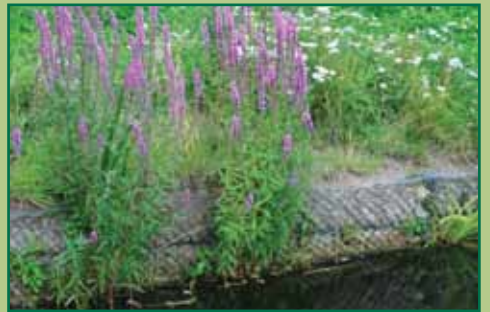
Vegetated coir rolls three months later.
